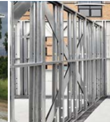
Structure de cloisons
